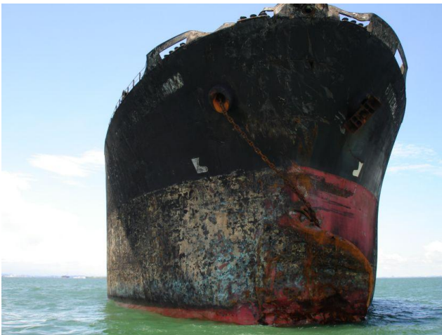
Ostende Max Fire and Structural Damage
