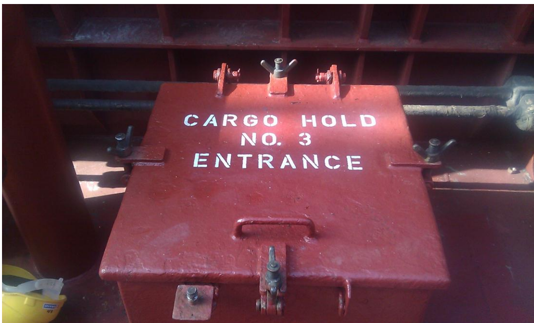
Entrance to Cargo Hold No.3 at the cargo recess area, located midships between No.2 and No. 3 cargo hatches (frames 95 to 101)
