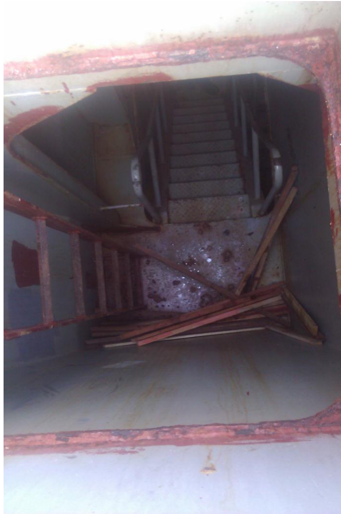
No.3 Cargo Hold Access showing Platform 1 at base of vertical ladder
