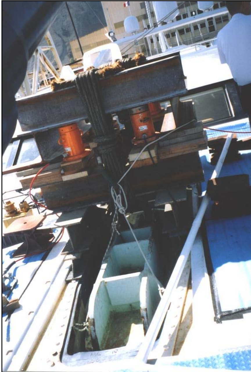
7. Temporary repairs made to keel lifting mechanism
