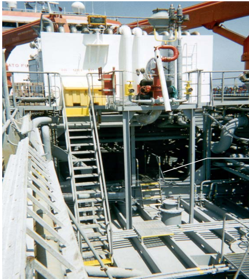
No.6 Centre tank lid
