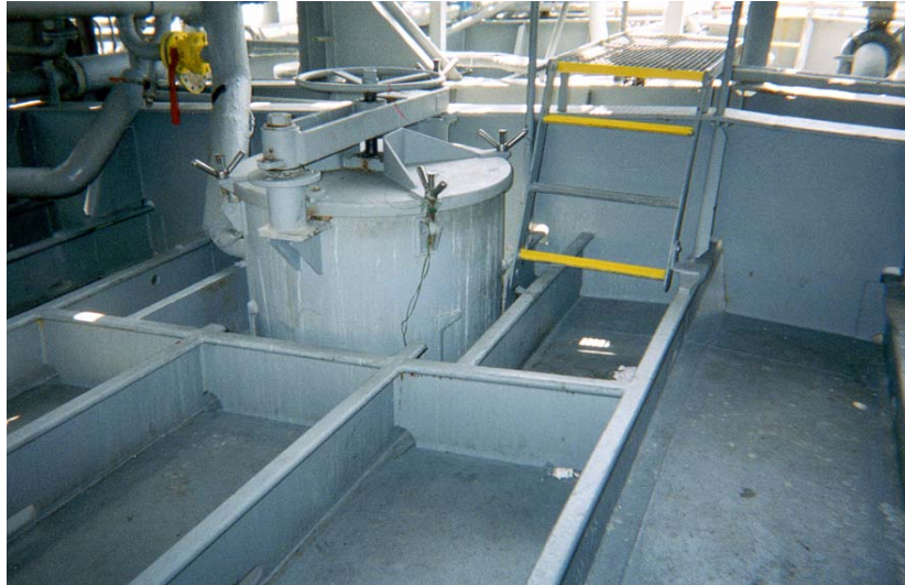
Photograph: Looking forward towards 6c tank lid. The warning notice of a Nitrogen atmosphere is attached to plastic wire on nearest tank hatch dog.
