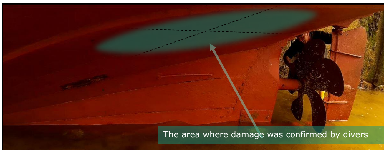
Figure 7/ Port quarter / May-2018 / The area where damage was confirmed by divers
