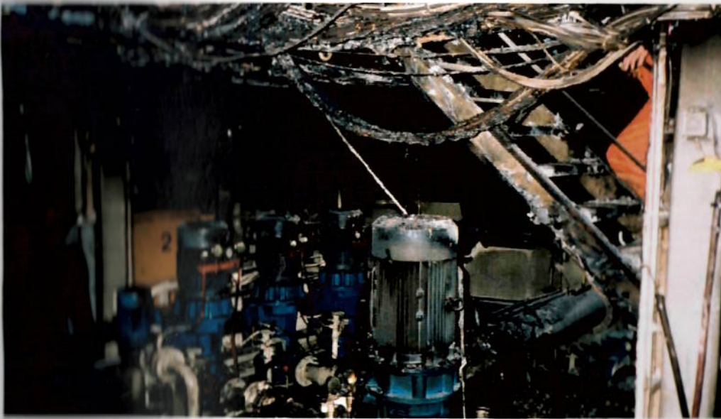
Fire damage to electrical fittings and wiring
