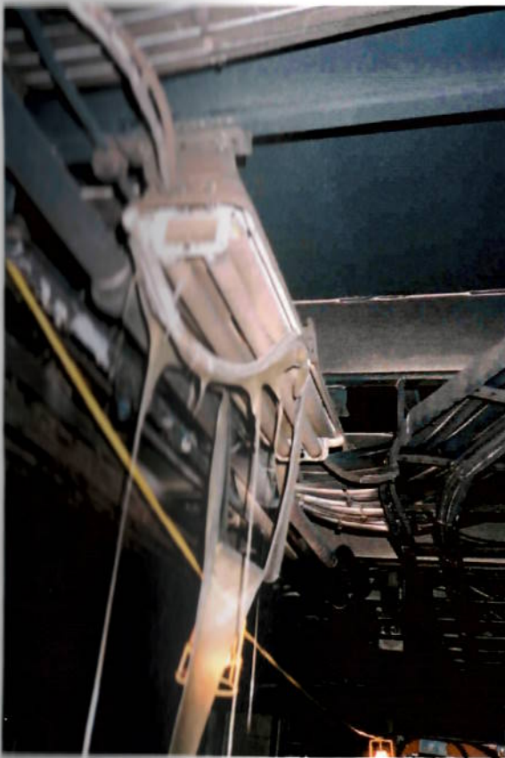
Fire damage to electrical fittings and wiring
